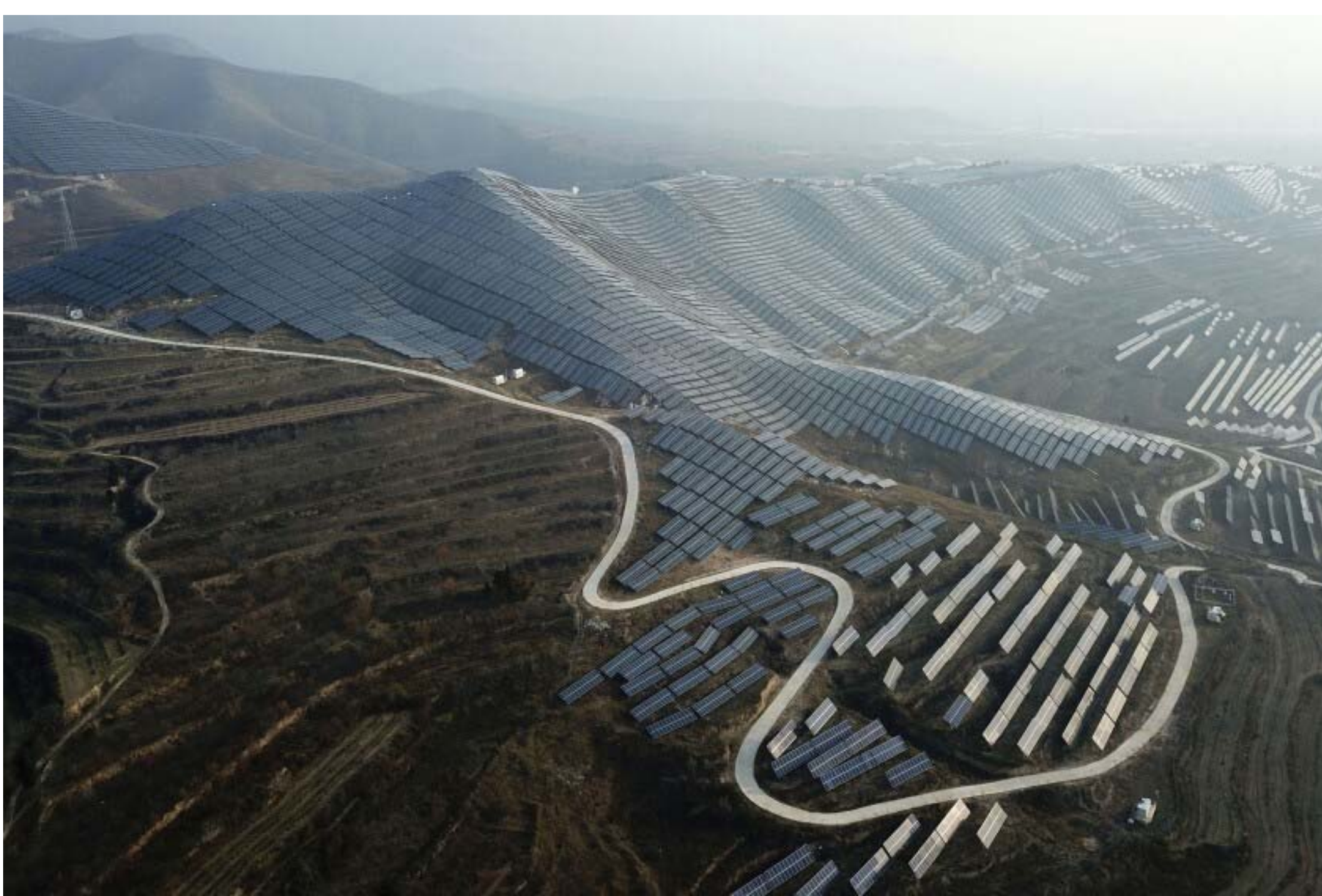
Solar panels blanket hills in China in 2019. (Sam McNeil / Associated Press)
